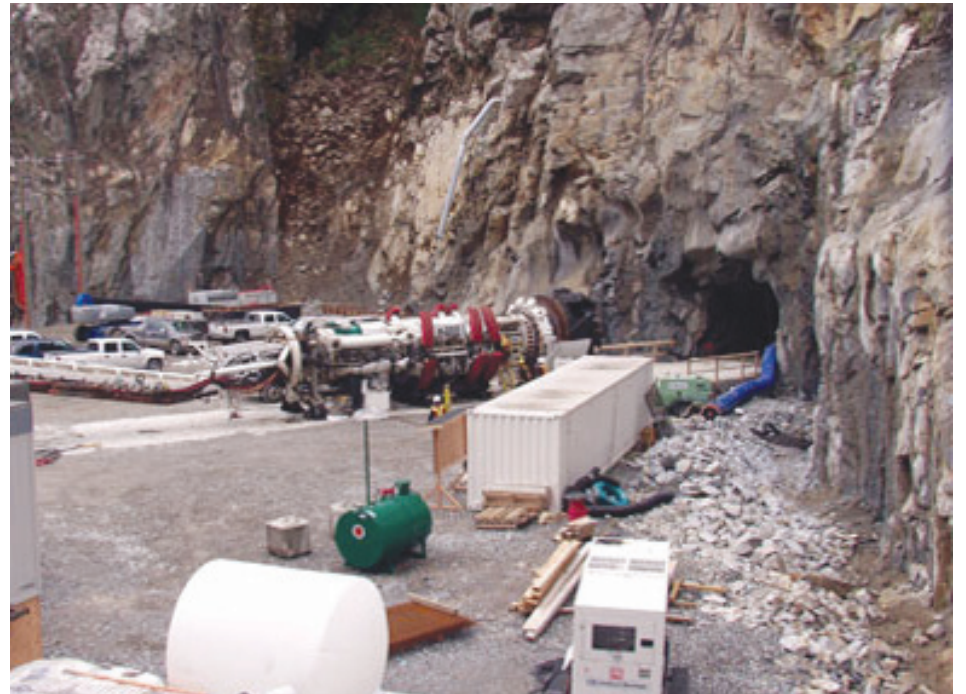
River-diversion tunnel at the Ashlu Private Power Project.
