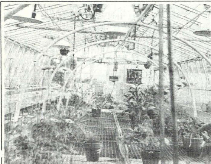
BCIT's existing greenhouse, located at the rear of the campus, will soon become part of a large complex. The structure will allow for more "hands-on" experience for students in the Biological Sciences technology.
