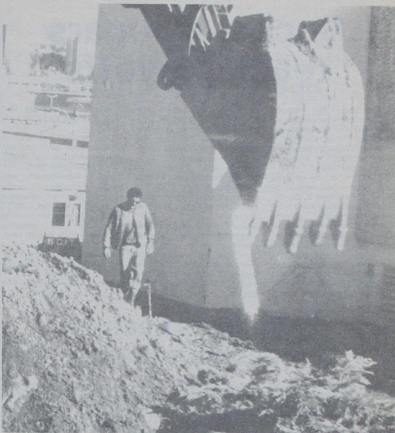
Men and machines work to repair drainage problem around Broadcast Centre. Plaster was falling off the walls of the building, letting water seep into
