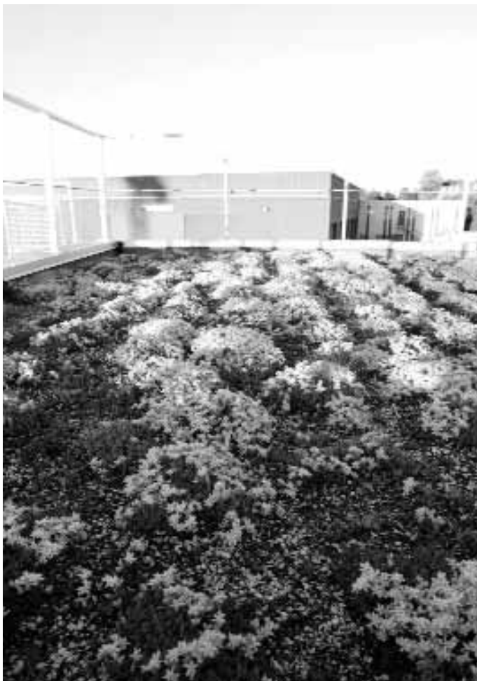
Green roofs like this one, at BCIT's Green Roof Research Facility, reduce storm water runoff and decrease a building's heating and cooling demands.
