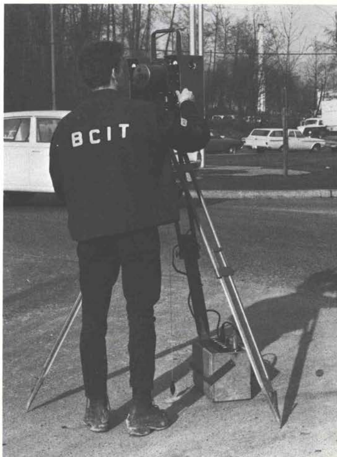
Surveying at work.
