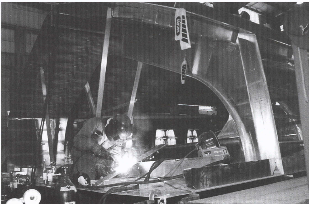
Welding inside the Fast Ferry
