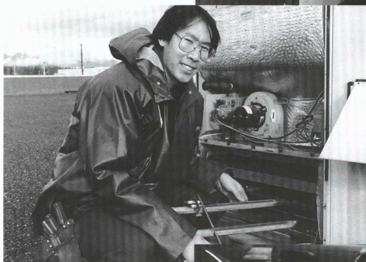
Lyle Cheng worked as an HVAC & R co-op student at Airstream Heating & Air Conditioning, where he is now an apprentice.
