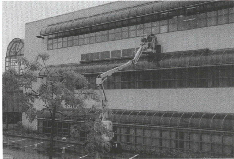
Faculty and staff from five different BCIT programs worked together to integrate a photovoltaic system into the building facade of the Tech Centre.
