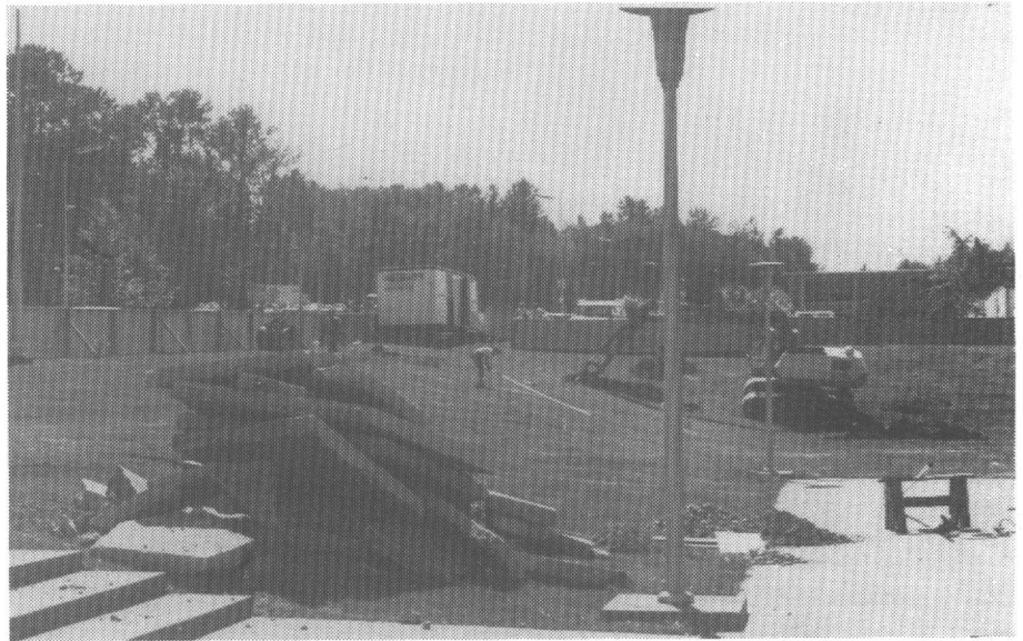
A backhoe digs trenches for sewer and electrical lines during groundbreaking for the new three-technology building to be located at the west end of the 1A '67 building.
